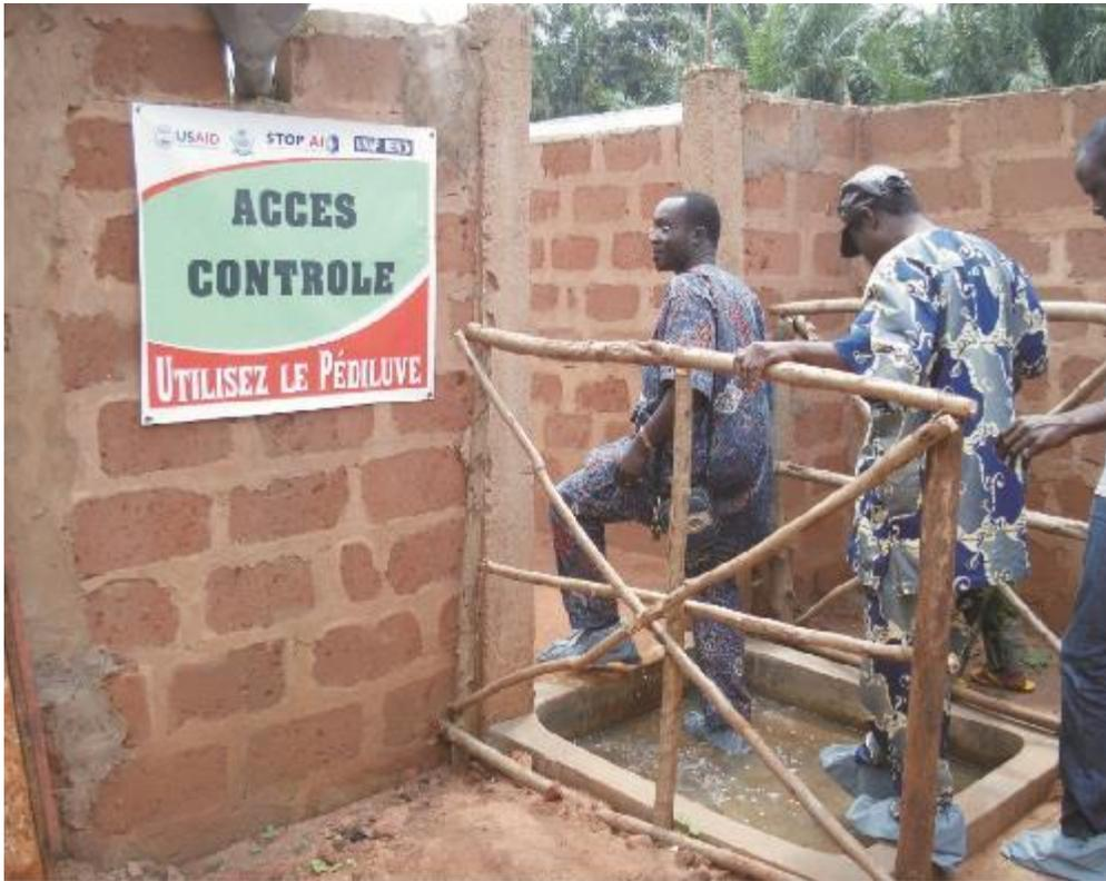
**Fig. 18: An effective but cheap foot bath at the entry to a poultry farm in Benin**
